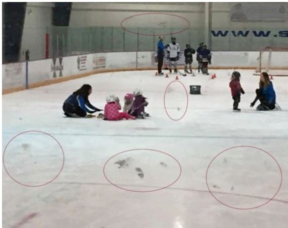
Figure 1. Puck marks on glass (circled in red) that obscure the view of spectators
